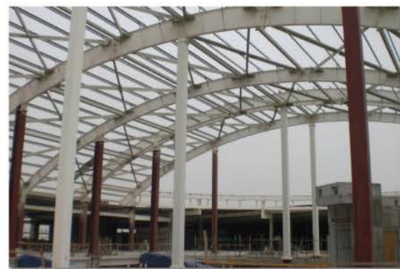
Curved Roof, Enma Mall, Bahrain
